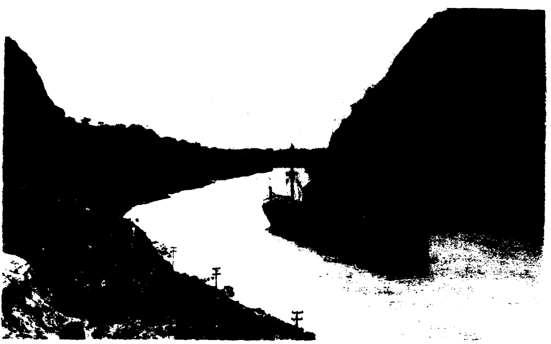
Ship passes through the Panama Canal at the Gaillard Cut, Cucaracha Slide, June 1921 Courtesy National Archives
