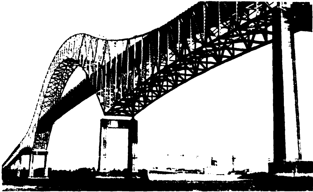
Thatcher Bridge over Panama Canal Courtesy Pan American Union
