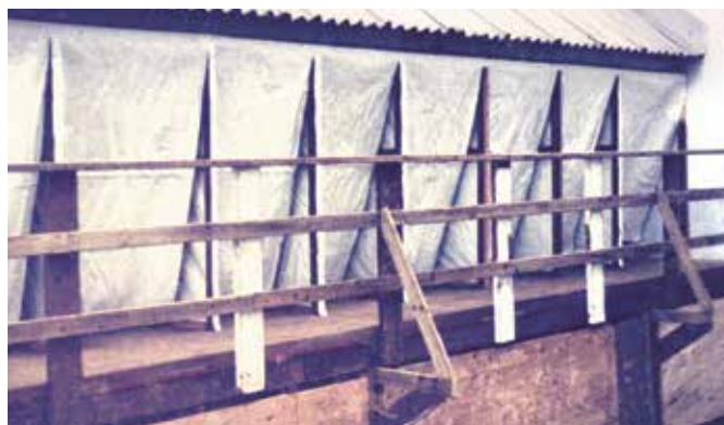
After engineers constructed toilets, MAJ Cheek had partitions and privacy screens installed.
