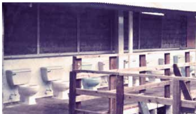
U.S. Army engineers installed commodes for the DCs’ use.
