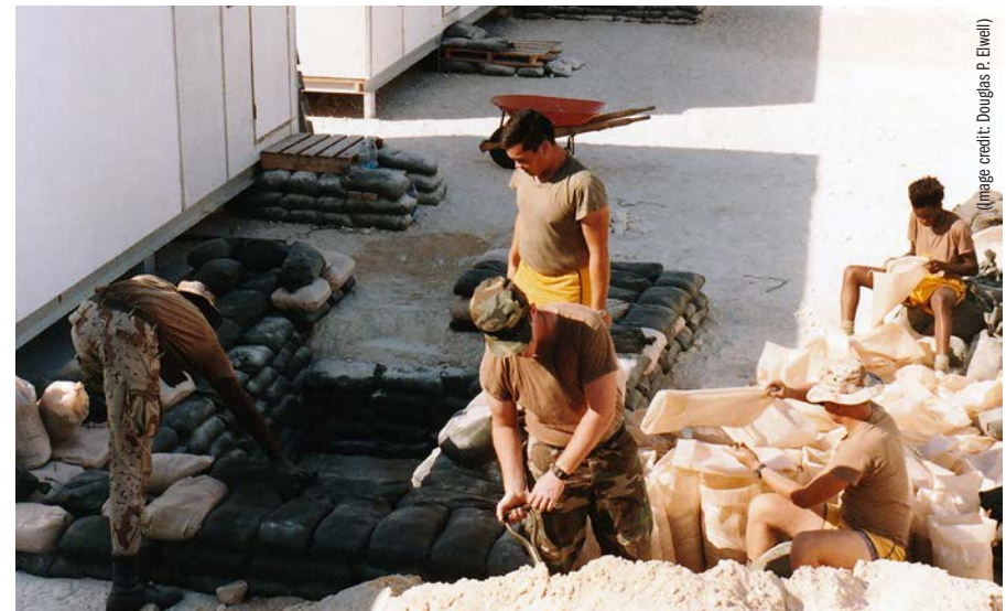
TOP: This photo was taken inside the PDB compound at KFIA, late 1990. The PDB was the only Army PSYOP unit permanently stationed at KFIA during the Persian Gulf War. BOTTOM: PDB soldiers fill sandbags for a bunker to protect against Scud missile attacks. As it turned out, within Saudi Arabia, KFIA would be spared from Scud missiles, unlike Riyadh, King Khalid Military City (KKMC), and Dhahran.
