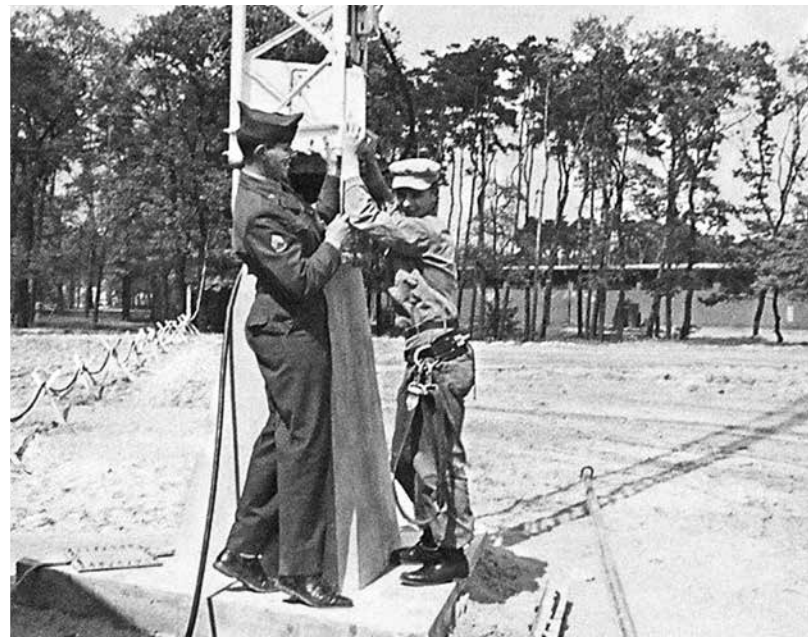
SSG Edward Berman and PFC Max Diamond of the MRBC stand at the concrete base of the 180-foot Gates Radio Company antenna that was transported overseas by 1LT Elmer R. Mosher, CPL Edward A. Mangold, and PFC Arthur J. Martin in early 1952.
