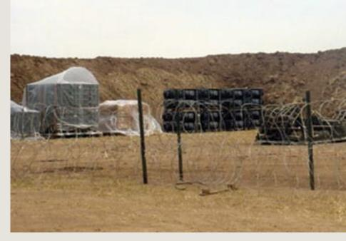
Under the supervision of Bravo FSC, Kurdish contractors built an Ammunition Supply Point (ASP) outside the base camp at Bashur Airfield near Irbil. A twenty-foot high berm surrounded the ASP, with six inner berms separating ammunition stacks. This ASP served special operations forces throughout northern Iraq.
