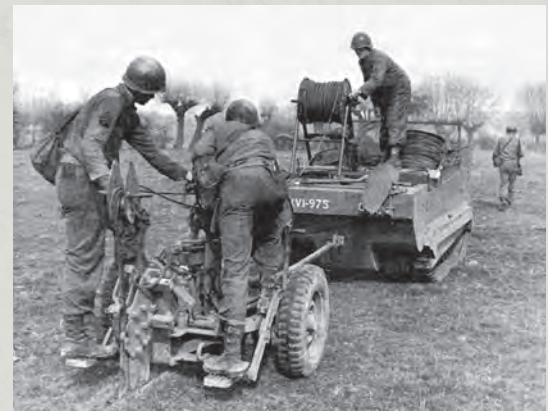
"Cable Dogs" of the 112th Signal Battalion burying communications cable to support the First Airborne Task Force (ATF) in Operation VARSITY, March 1945. The 112th soldiers parachuted across the Rhine to provide communications support. The 112th later established the 1st ATF communications network during the link-up with the Russian Army on the Baltic.
