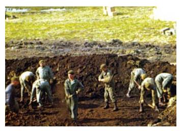
In order to pitch their Bell tents in the tundra, the Forcemen rolled back the muskeg and dug down to the volcanic bedrock. They drove their tent pegs into the rock to hold the tents up in the nearly continuous heavy winds.
