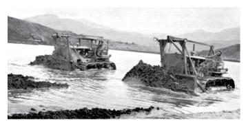
Bulldozers dredging sand from Adak inlet to use as fill for the new airstrip. The ability of the U.S. forces to construct airfields in the Aleutians was a major factor in defeating the Japanese forces on the islands.
