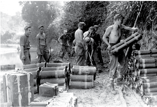
The Field Artillery received its ammunition in clover-arranged tubes of three, that were packed three to a mule. Each gun had at least a basic load of twenty-seven rounds at all times.
