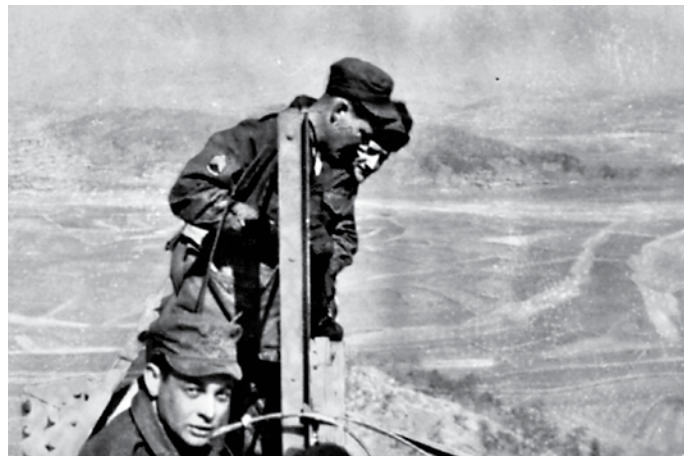
A good "head for heights" was a prerequisite for the riggers who repaired the Korean Broadcasting System antennas and erected the antennas to support the 4th Mobile Radio Broadcasting Company operations.
