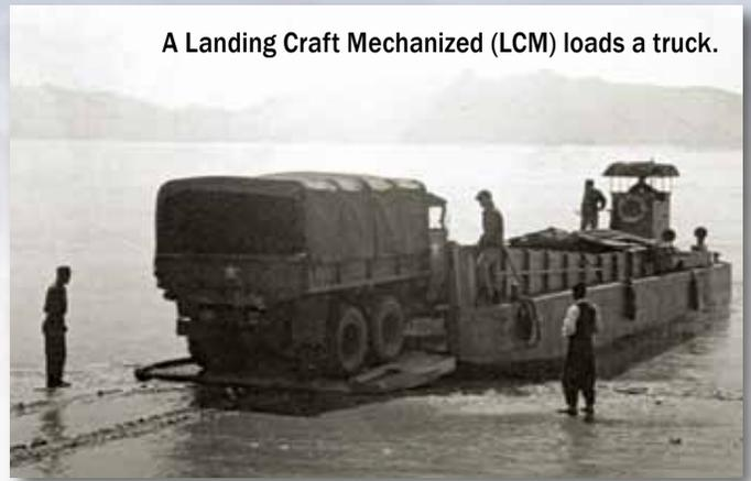
A Landing Craft Mechanized (LCM) loads a truck.
