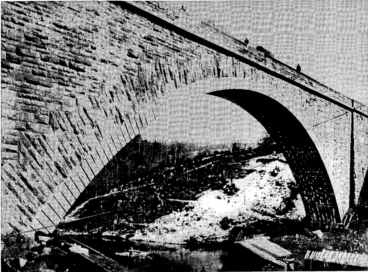
Another major U.S. Army project, the renowned Washington Aqueduct. Signal Corps, National Archives
