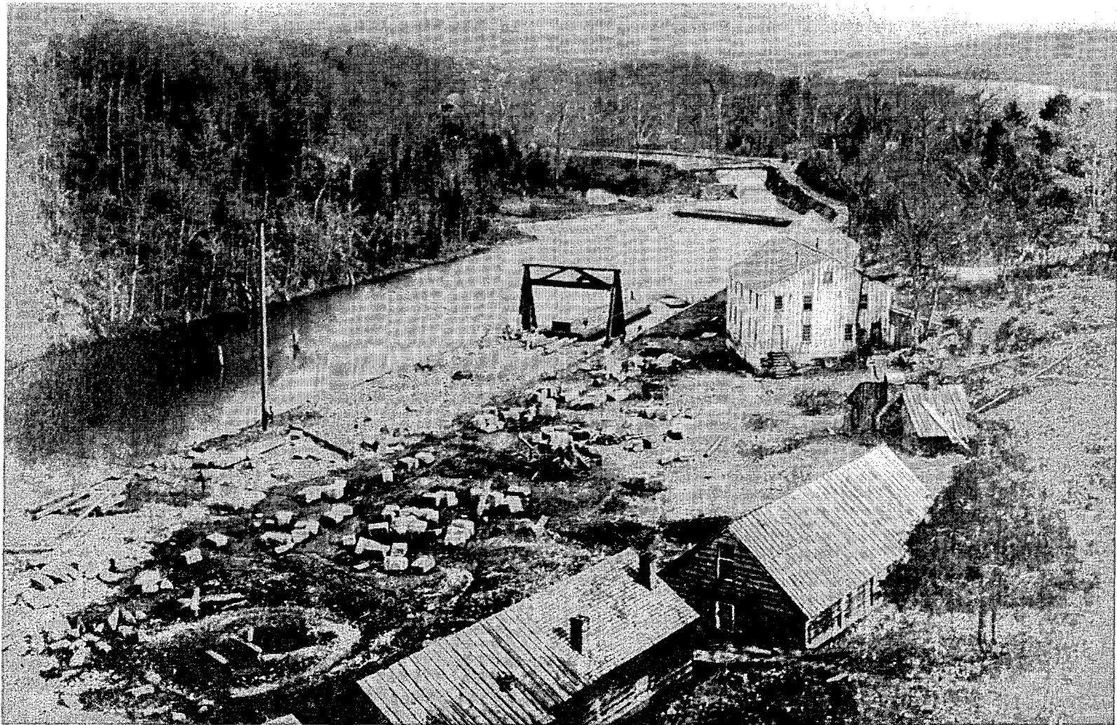
U.S. Army "nation-building," the Chesapeake and Ohio Canal under construction. An engineering marvel but a financial failure, losing out to the railroad. Signal Corps, National Archives
