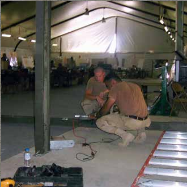
Construction of the large utility tent housing the Joint Operations Center (JOC) and other office spaces.
