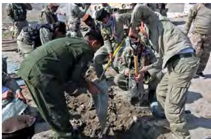
Afghan Local Police (ALP) fill sand bags during the construction of a traffic checkpoint in Jegdalay district, Kabul Province, Afghanistan, 5 March 2014. ALP assisted by U.S. Special Forces soldiers assigned to CJSOTF-A. The checkpoint disrupted insurgent freedom of movement. DoD Photo
