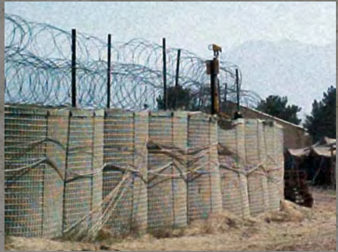
Photo showing a portion of the HESCO perimeter wall around the CJSOTF Headquarters in April 2002. Note the addition of lighting for night operations. Surveillance cameras were installed to allow guards to remotely view sectors without exposing themselves to direct fire weapons.
