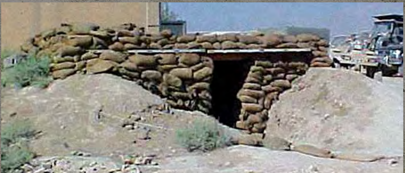
Expedient bunker to provide protection from indirect fire attacks. Over time, these were replaced with above-ground concrete and sandbag bunkers. In those early days the troops experienced random direct fire attacks which were gradually replaced with sporadic monthly indirect rocket or mortar attacks.
