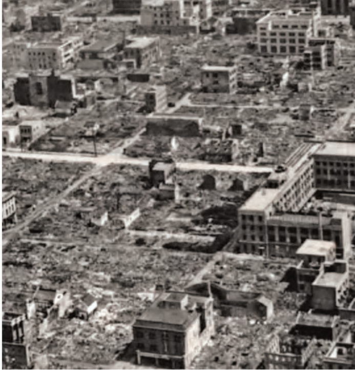
The Japanese city of Osaka suffered greatly from the U.S. bombing campaign. One of LTC Munske's duties was to help restore services to the damaged city.
