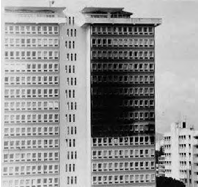
Post-mission photo of the target building, the smoke damage from the fire is clearly visible.
