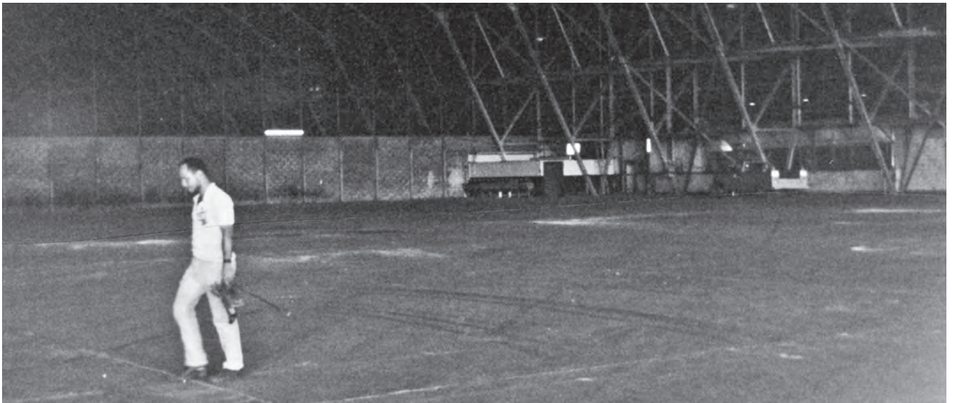
Top: This view shows some of the vehicles that were parked in the hangar. MAJ Cheek directed their removal so he had space to create a DC shelter. Middle: A second story office inside the hangar provided a place for facility employees to work once the camp was up and running. Previously, it served as MAJ Cheek's office. Bottom: When U.S. Army engineers removed the vehicles, weapons, and ammunition, MAJ Cheek directed that the hangar be cleaned. Once clean, Panamanian laborers began construction of individual housing cubicles.
