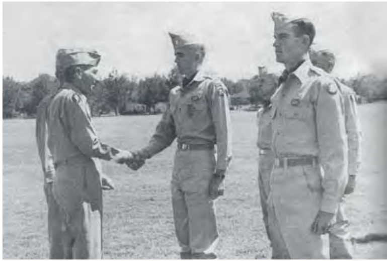
First Lieutenant Ralph Puckett Jr. is awarded the Distinguished Service Cross at Fort Benning, Georgia.
