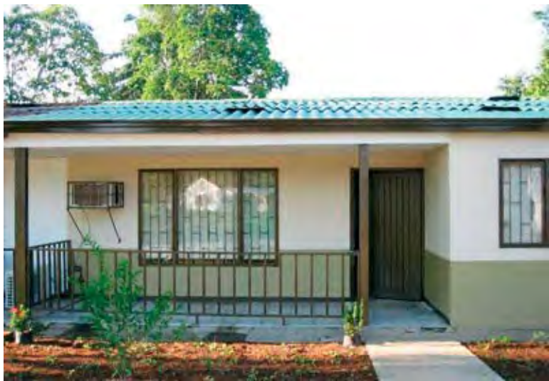
PATT facility in Villaviciencio, Colombia, sixty kilometers south of Bogotá. The quality of PATT housing varies widely.
