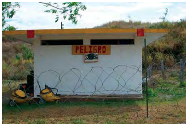
The small out building at serves as the ammunition supply point at Pijaos.
