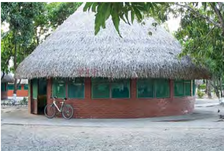
A typical classroom building used at the CNP training center in Espinal.
