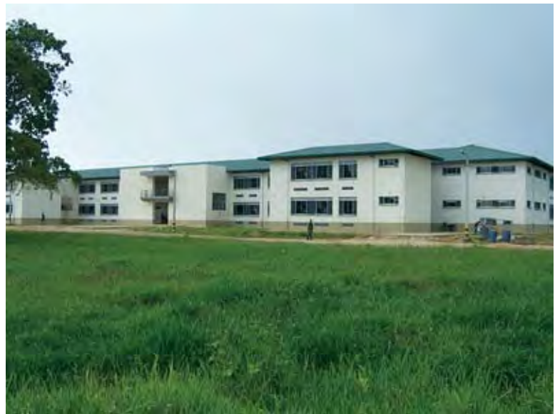
View of one of the new barracks built at Larandia using Plan Colombia funds.
