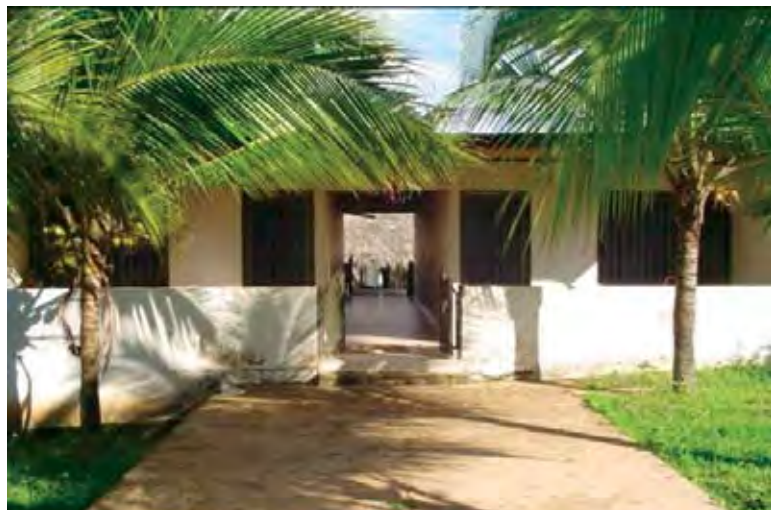
The FARC built extensively throughout the despeje (sometimes called “FARClandia” by the Special Forces). This is a house used by one of the higher FARC leaders.
