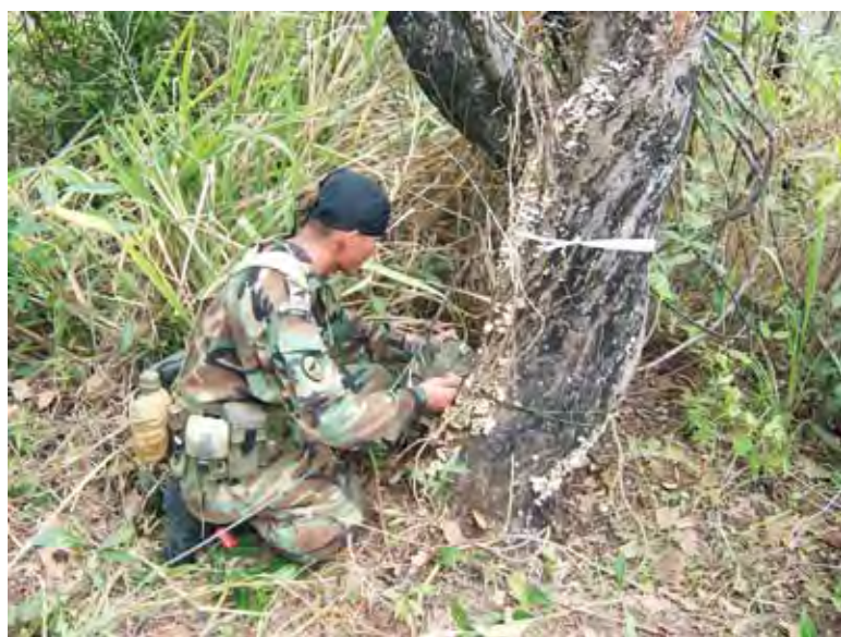
A Colombian special forces soldier sets charges on a tree. One challenge is to use just enough to clear the tree and not waste explosives.
