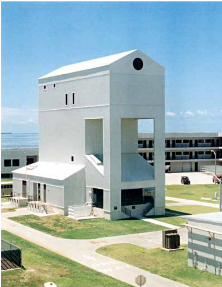
The new fifty-foot dive tower allows for the simulation of locking out of a submarine and for training in the free ascent from deep water.
