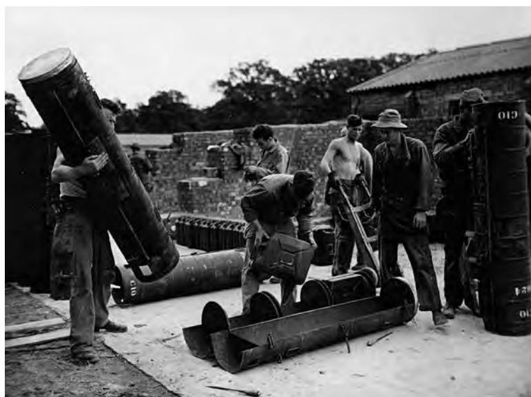
Gasoline being packed in type "C" containers. Notice the brick revetting walls.
