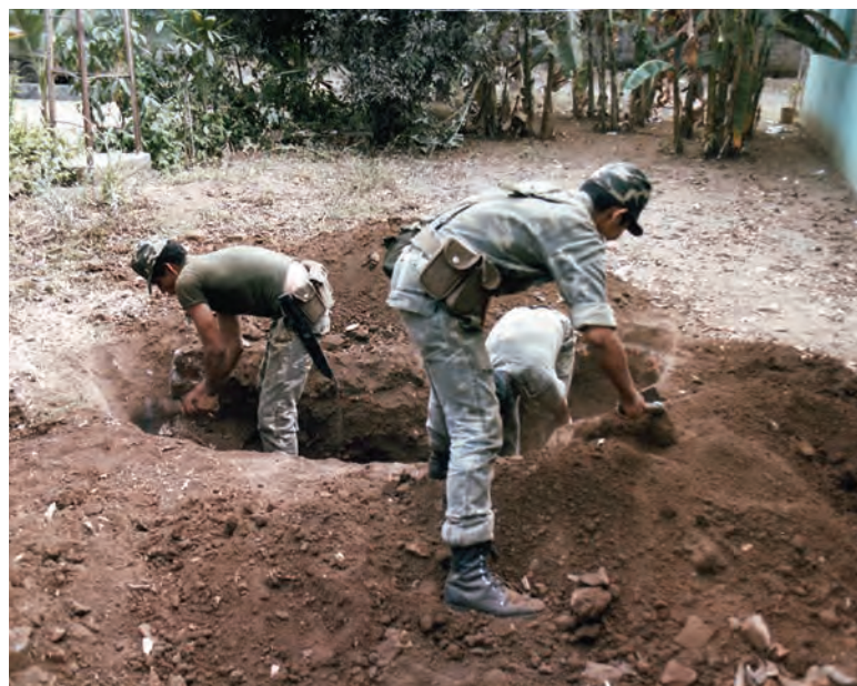
The primary digging tool for the ground defensive positions was the U.S. Army folding entrenching tool. The rock-hard dirt was used to fill the sandbag barriers in front of each position.
