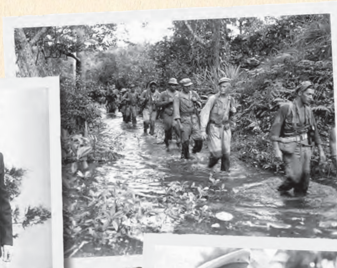
Alamo Scout training was arduous and intensive, concentrating on reconnaissance techniques and honing the men's ability to move through the jungle. Here trainees at the ASTC at Kalo Kalo conduct a forced march on Fergusson Island, New Guinea, February 1944.
