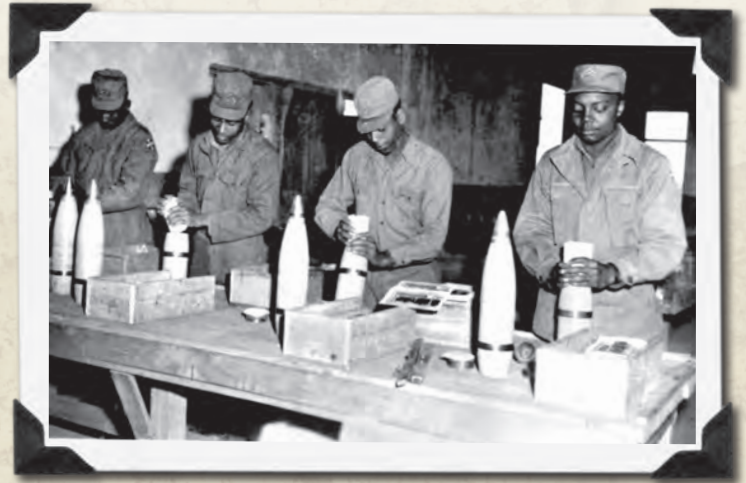
Leaflet rolls being loaded into 105 mm Base Ejection (BE) Smoke shells at the EUSA Ammunition Supply Point (ASP) prior to being shipped to Corps artillery units.
