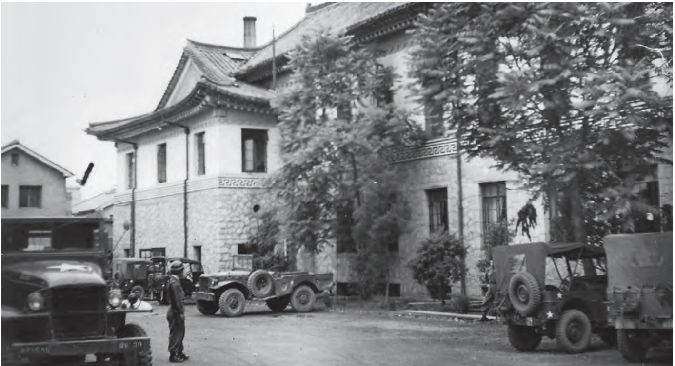
8240 th AU Headquarters in Seoul was a Presbyterian mission school. Living quarters were located on the second floor.
